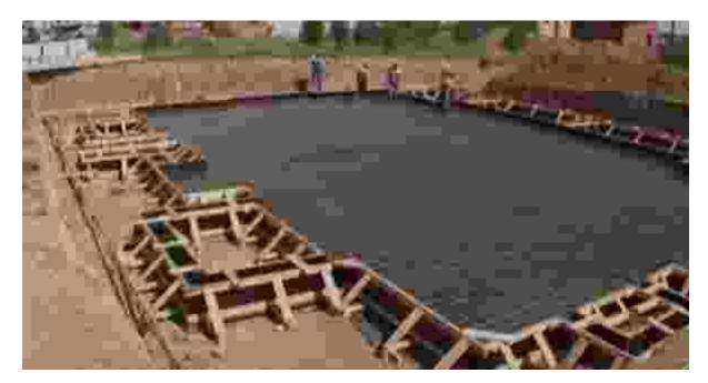
Figure 3: Compensated raft foundation under construction
