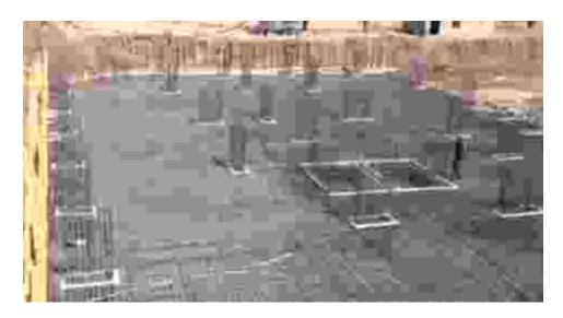
Figure 1 Raft foundation under construction
