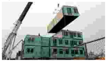
**Figure 10:** Image showing an ongoing prefabrication construction process **Source:** Farid (2019)
