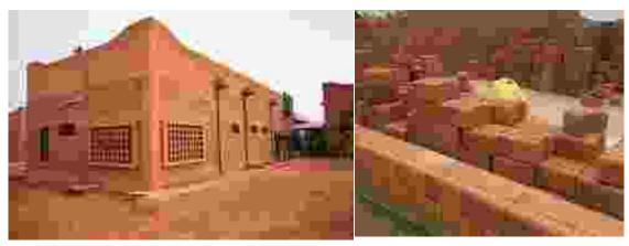
**Figure 9:** A typical compressed earth block building **Source**: *Kaitlin (2017)*.
