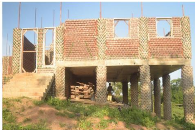
Fig. 2: Multistorey building construction building with eco-bricks
