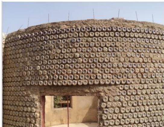
Fig. 1: Single storey building construction with eco-bricks
